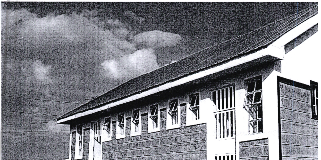
Njiru Secondary School Ablution block
