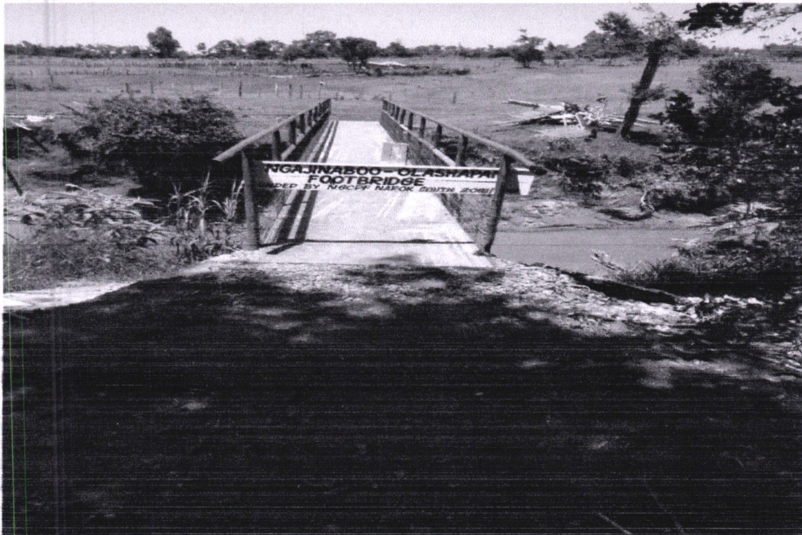
OLE NKAJI NABO FOOTBRIDGE FUNDED BY NAROK SOUTH NGCDF 2018/19
