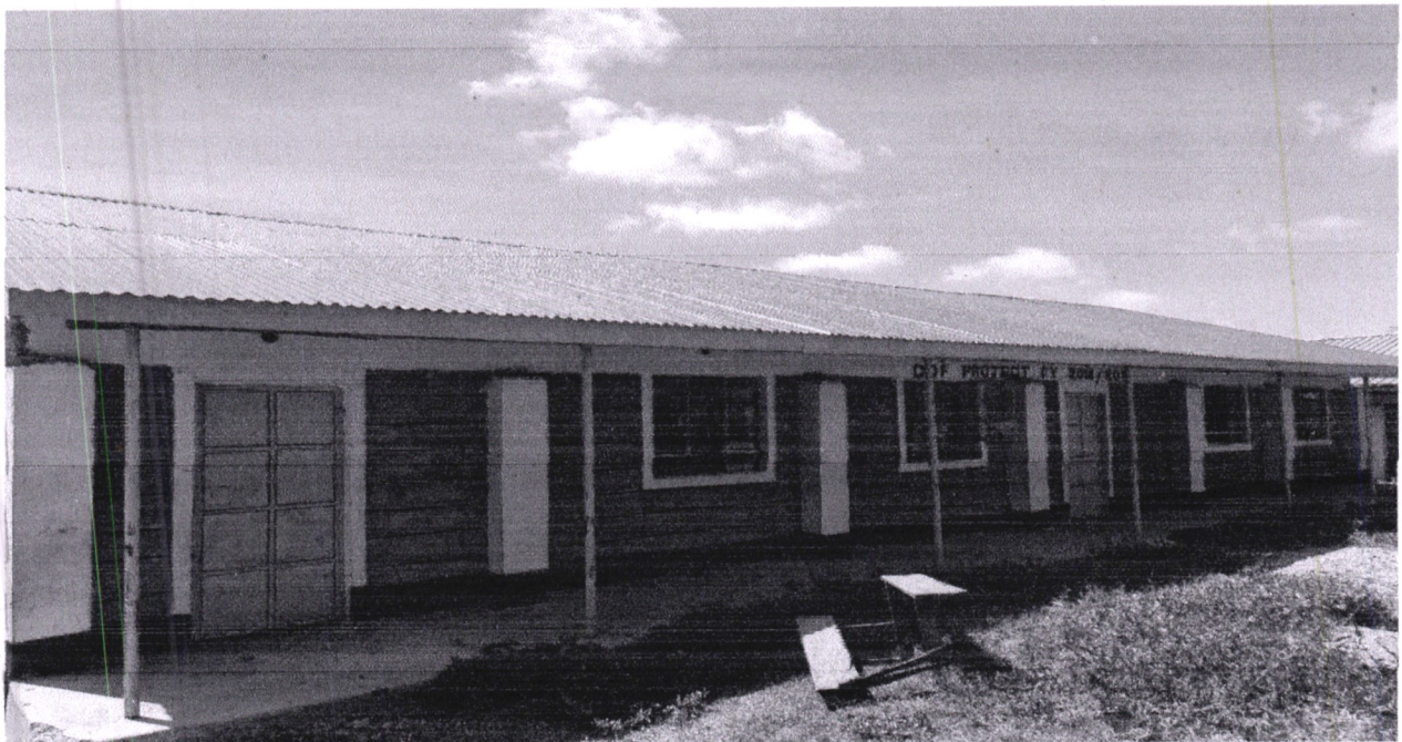
OSINATEI PRIMARY SCHOOL-TWO CLASSROOMS FUNDED BY NAROK SOUTH NGCDF 2018/2019
