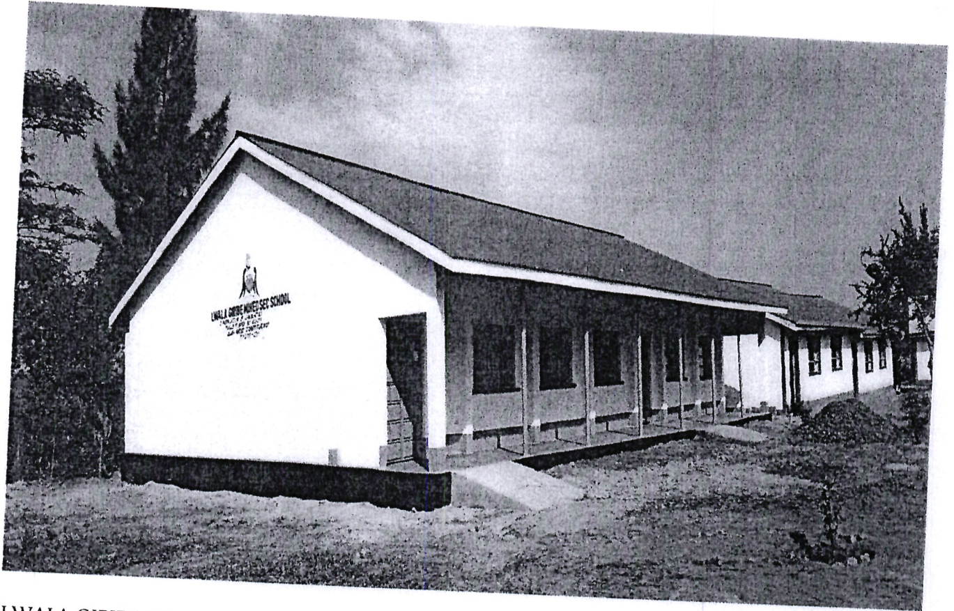
LWALA GIRIBE MIXED SECONDARY LABORATORY CONSTRUCTED BY SUNA WEST NGCDF
