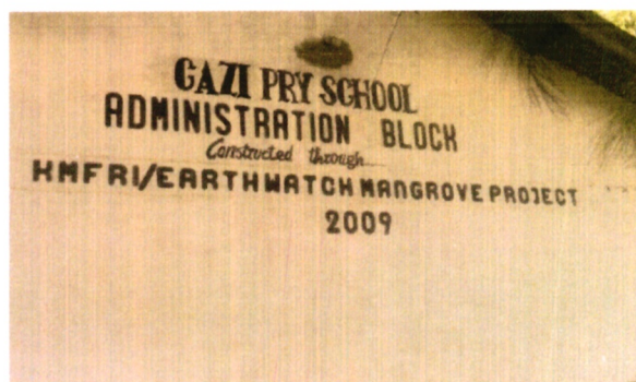
Figure 2: Photo of the administration block constructed by KMFRI/Earthwatch project
