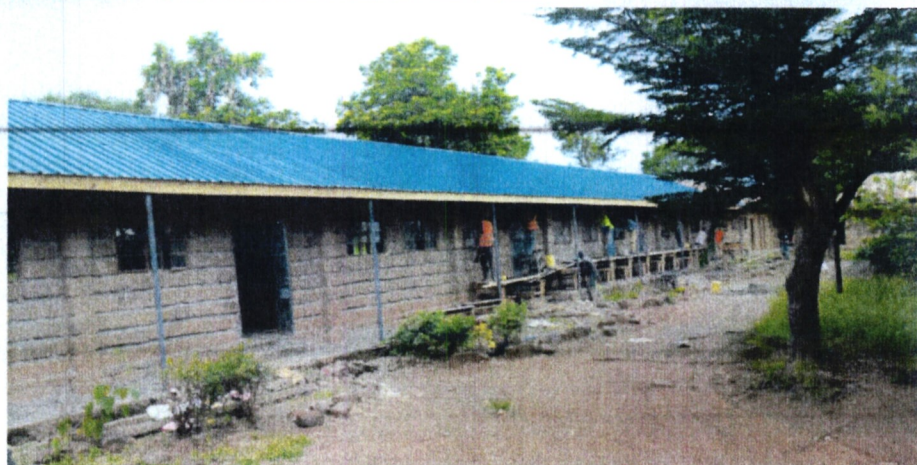
Above: Renovation of 4 classrooms at Ruiru Primary School- project ongoing
