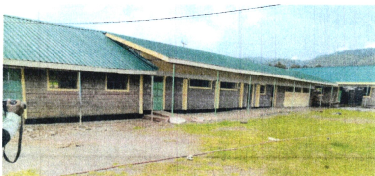
Above: Endao Primary School-Construction and Renovation of Classrooms
