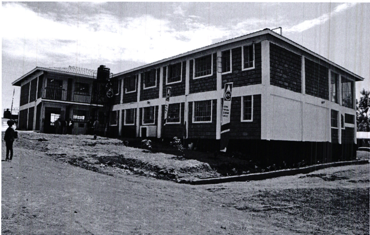
Construction of 4No.classrooms 1 storey block at Cheptuiyet Girls High School was done by KPC Foundation.
