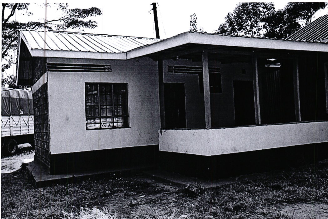
Kihoya Ass/chief's office Project Activity: Renovation of Ass/chief's office
