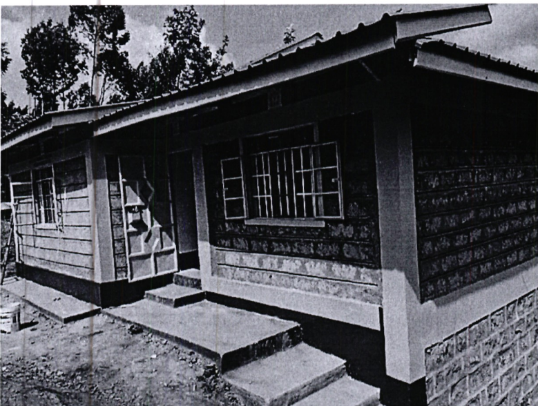
Githima Primary School Construction of administration block
