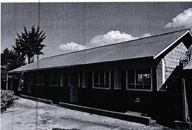
St Johns kiruri primary school Construction of 2NO. classrooms
