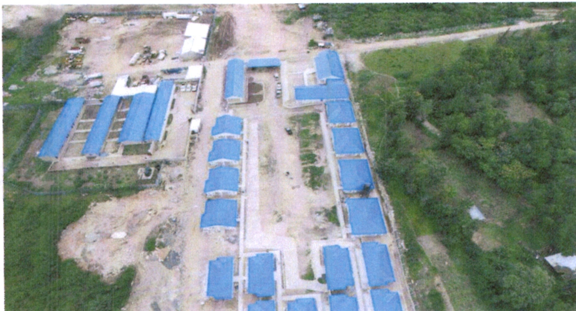
Completed construction of RE's Offices, Residence, Labs & Contractor's camp
