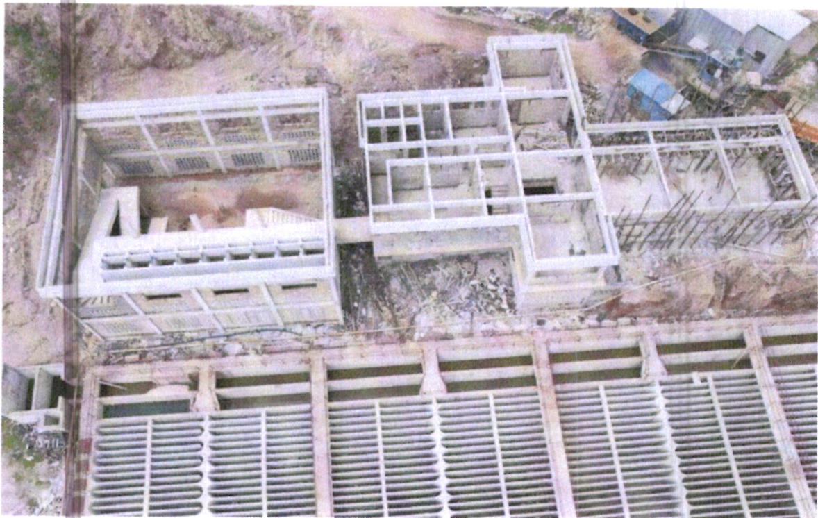
Ongoing works at the Water Treatment Works at Kabichbich
