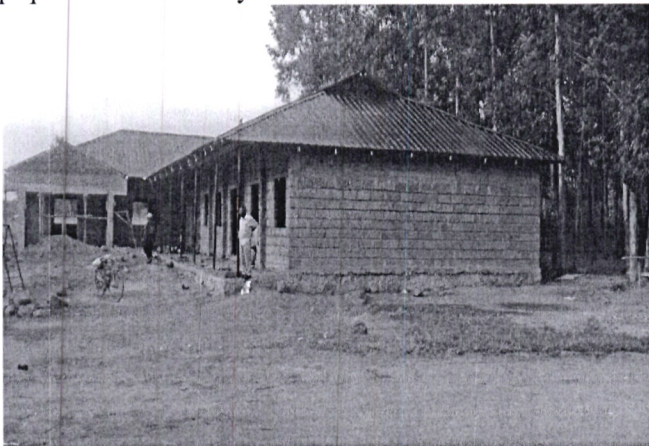
PHOTO OF NAPARA ACK CLASSROOMS UNDERCONSTRUCTION
