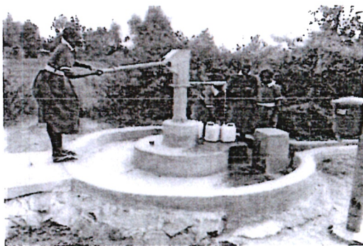
OKATEKOK BOREHOLE IN OPERATION
