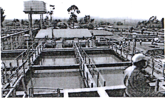
REHABILITATION OF TREATMENT WORKS BY THE COUNTY
