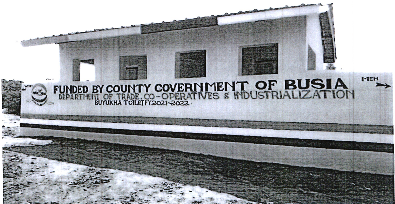
Toilet building at Bukhuya market
