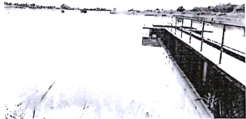
Busia Sewerage Treatment Plant
