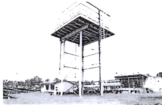
400 CUBIC STORAGE TANK- MUNDIKA WATER WORKS
