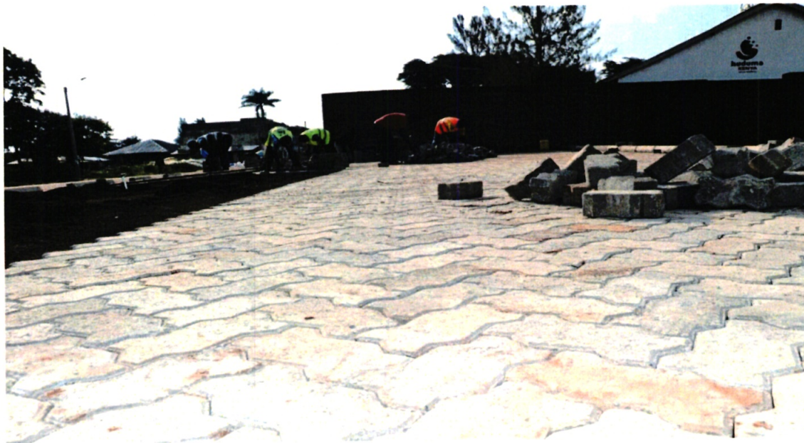
Construction of parking lot in Busia town adjacent to Huduma centre
