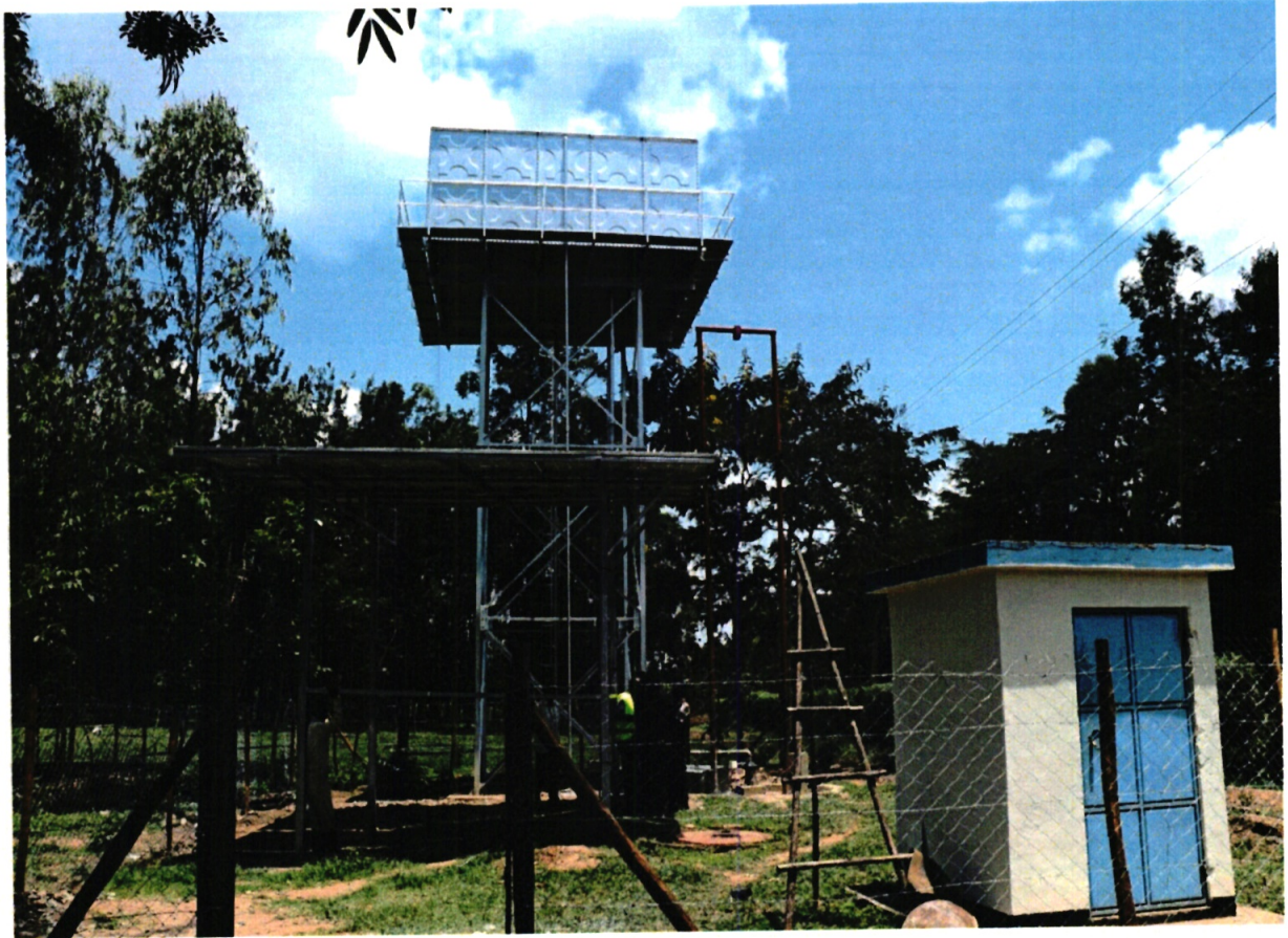
The County drilled several boreholes across the county
