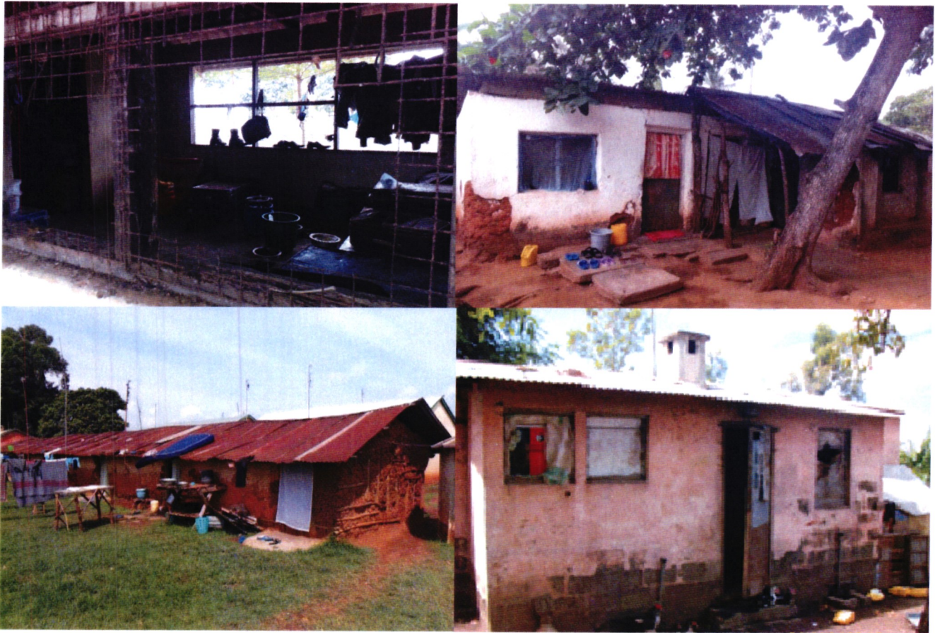
Plate 4: Samples of dilapidated residential houses as observed during the audit
