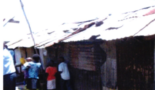
v) Iron sheet house (Nairobi Remand)
