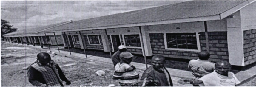
Korokou Girls Sec.school Two Classrooms
