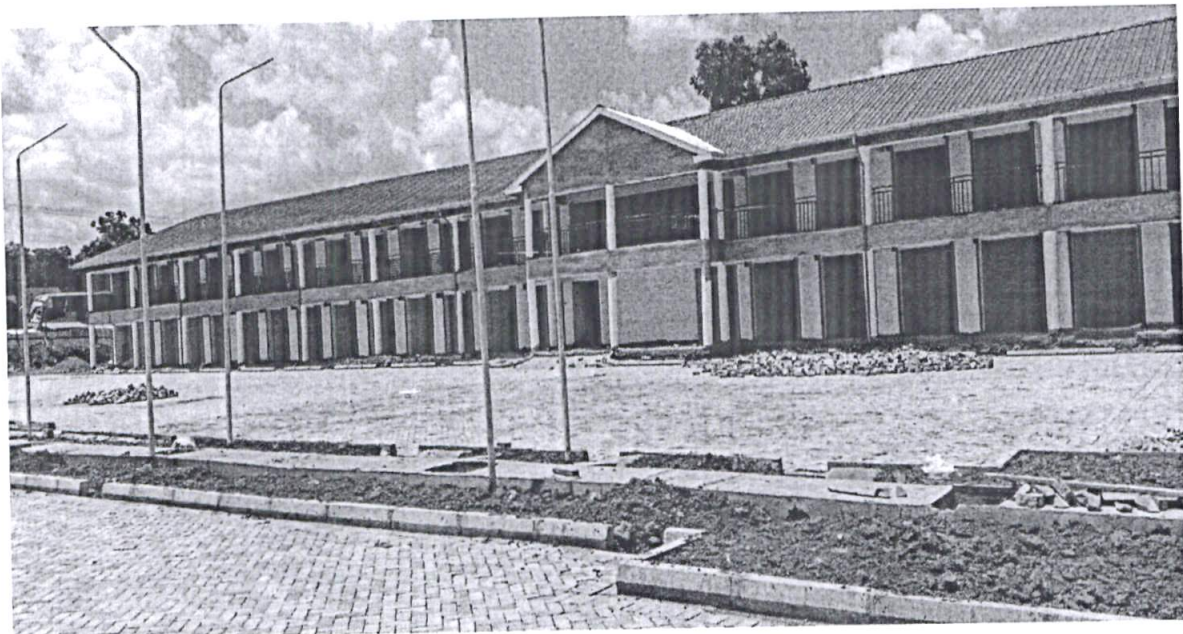
Figure 4: Modern bus park in Kanduyi
