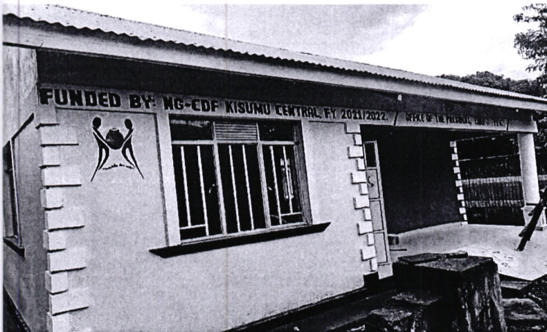
Construction of Southern Sublocation-Assistant chiefs office
