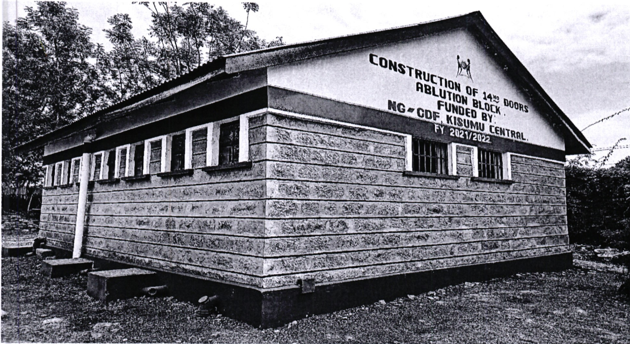
Lions High School-Construction of Ablution Block
