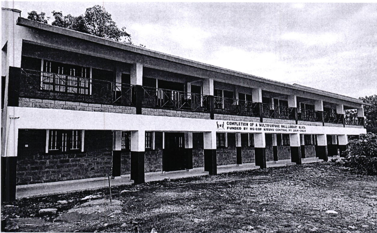
Joel Omino Secondary School-multipurpose hall/library block
