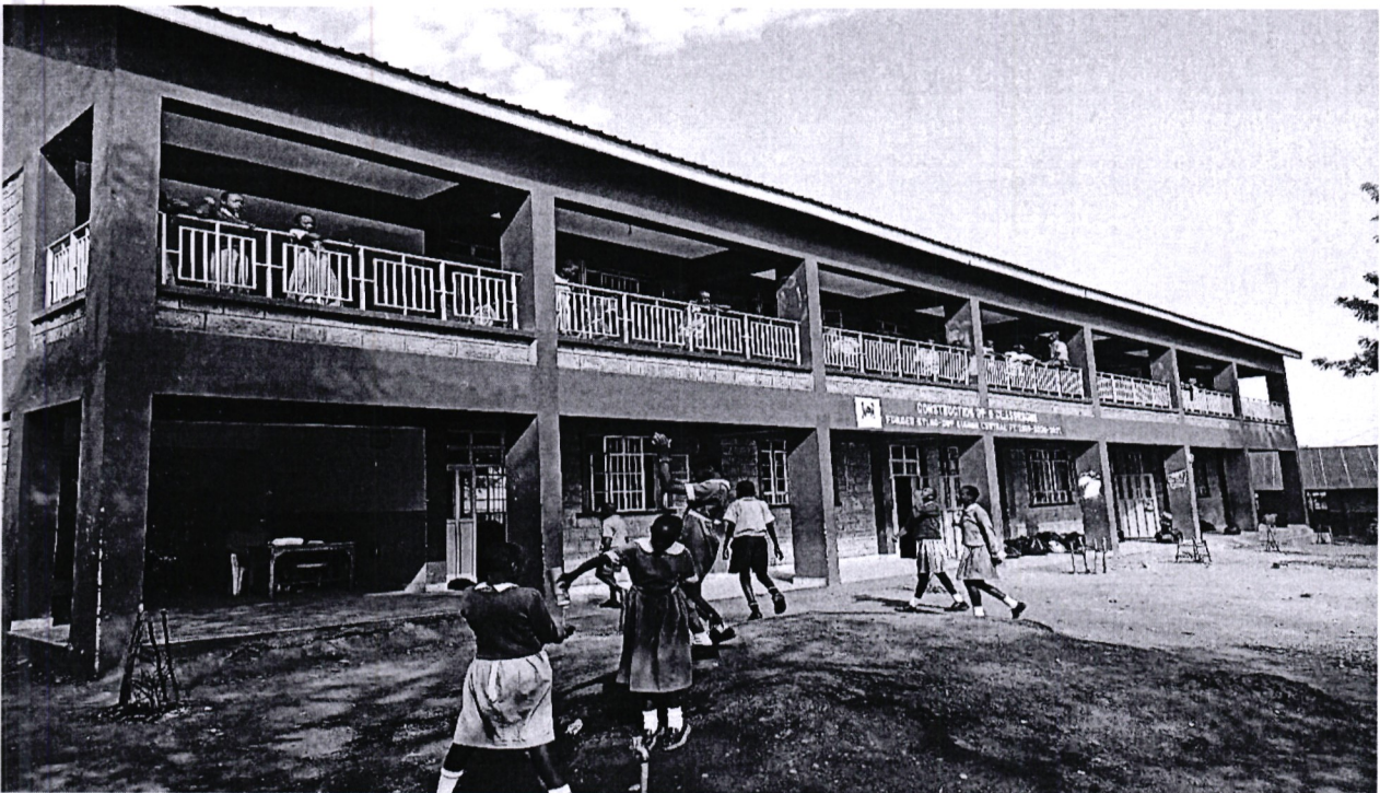
Construction of a storey building made of 6no. Classrooms at Obinju Kanykavar Primary School
