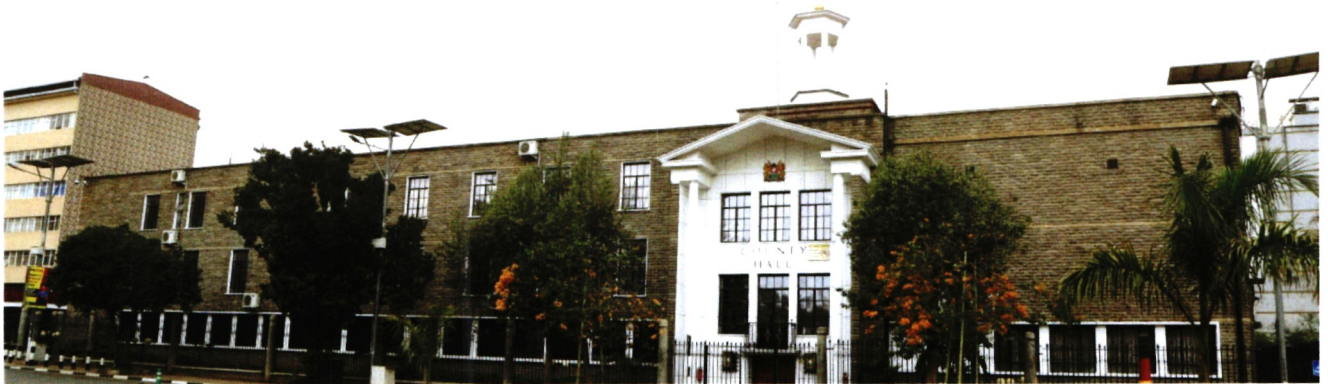
County Hall Building - the home of Parliamentary Service Commission
