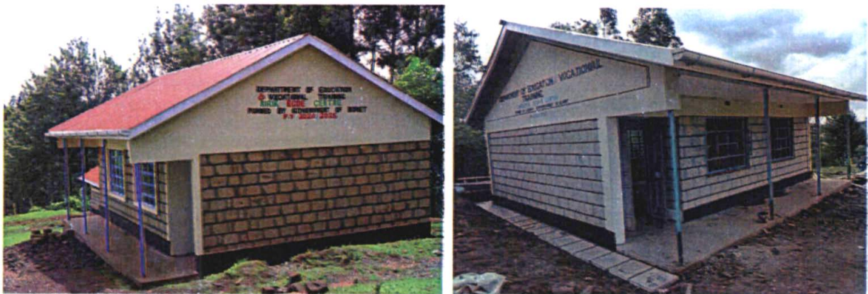
Fig. 1 Completed ECD classrooms
