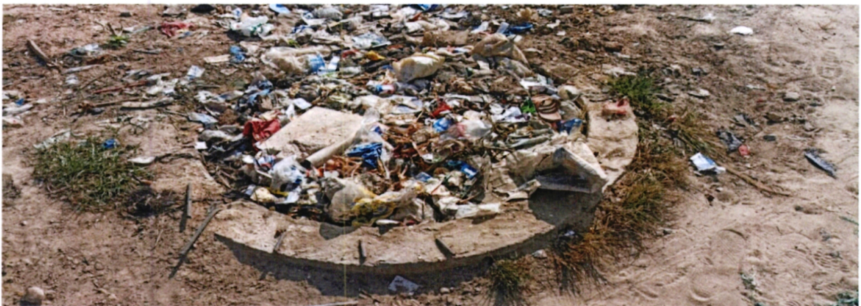
One of the manholes constructed under the Changamwe Re-pooling Secondary Sewer Project turned into a dumping site (photo taken on 23 January, 2025 by OAG auditors)
