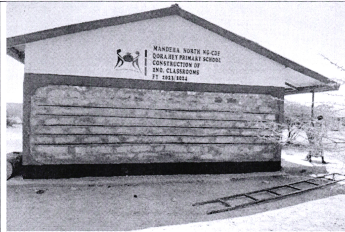
QORAHEY PRIMARY SCHOOL CONSTRUCTION OF 2NO. CLASSROOMS FY 2023/2024
