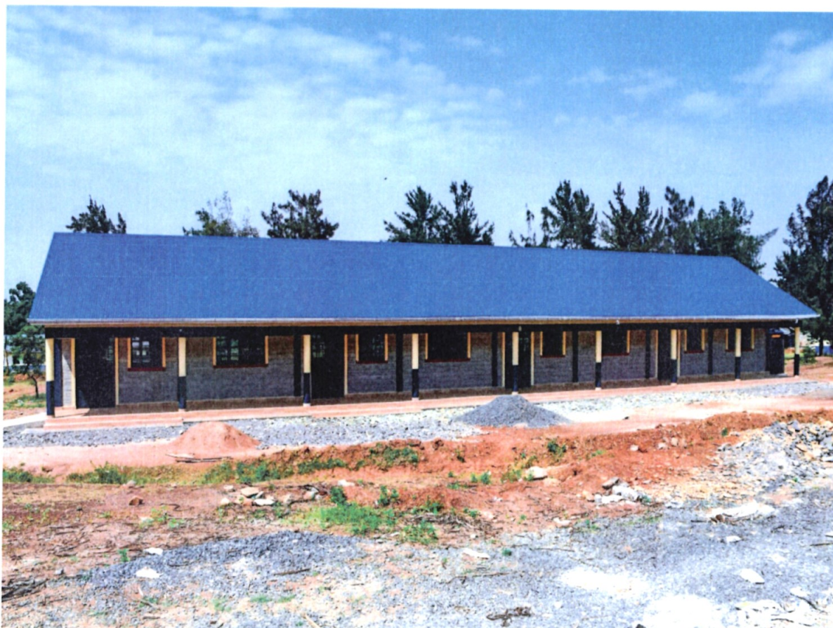
Construction of 4no Classrooms at St Pauls Kanyakwar Comprehensive School
