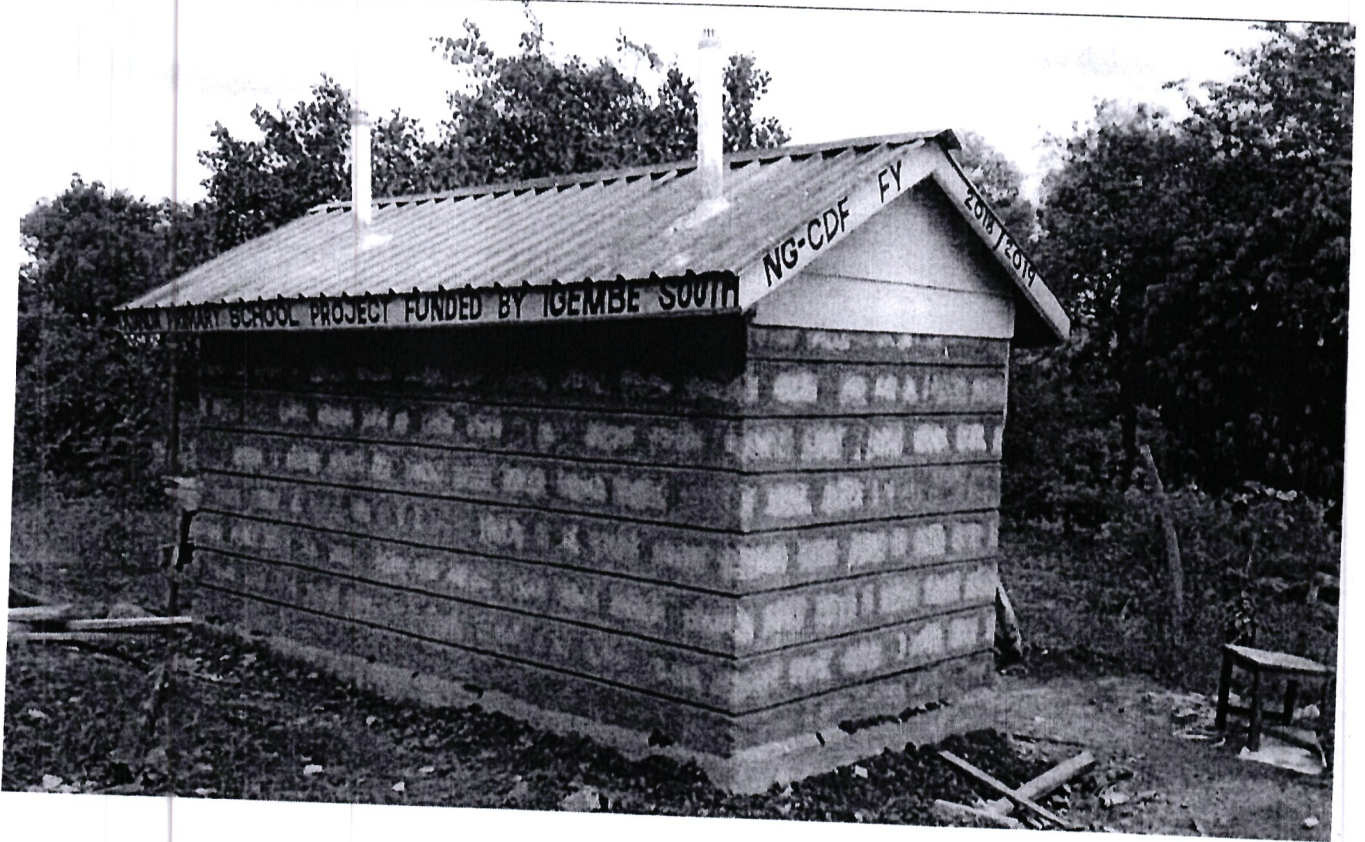
Kianda primary school pit latrines
