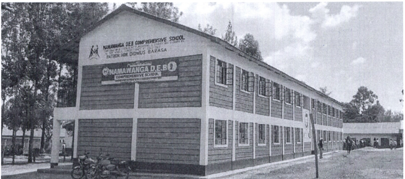
Fig 4: Completed one storey building 8 No. Classrooms at Namawanga DEB Primary School
