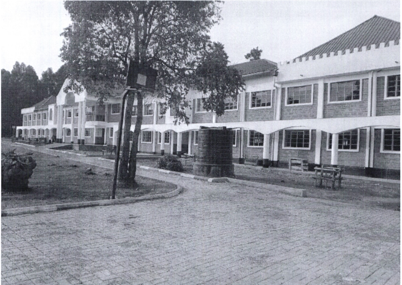
Fig 3: Completed one storey building 16 No. Classrooms and administration block at Kamukuywa AC Primary School
