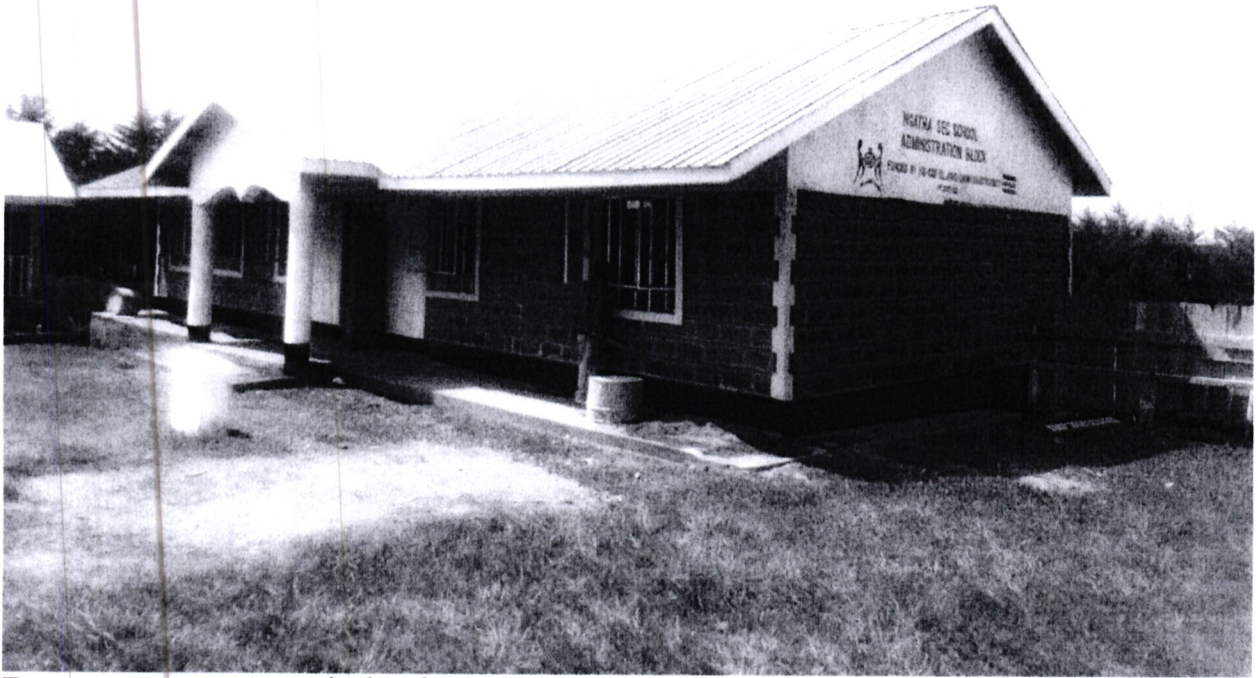
Due to emergence to lack of security for school documentation, we constructed a schools administration block at Ngatha secondary school as shown in the above diagram in charagita ward.
