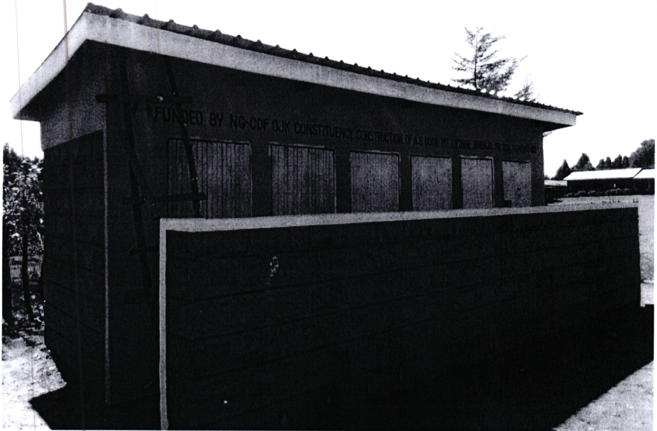
Due to High Need of Education and population, we constructed a six door pit latrine with urinal at Mwenja primary school to enhance hygiene as shown in the above diagram in Gathanji ward.
