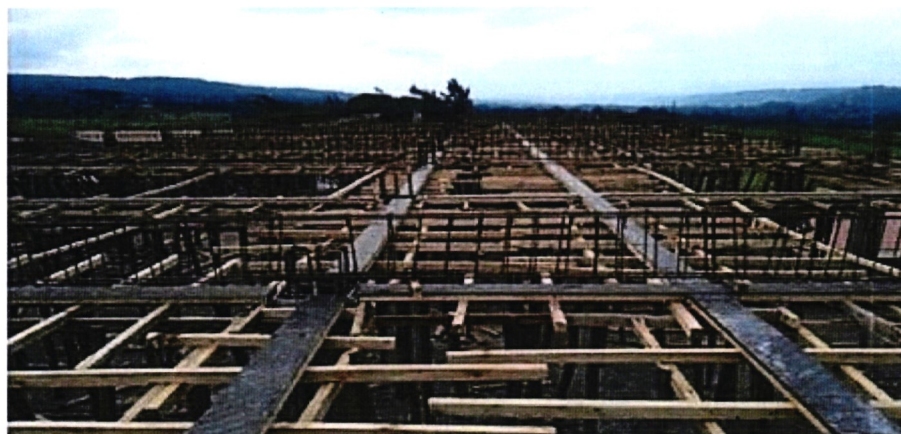
BLOCK B FINAL RING BEAM TO SUPPORT ROOF
