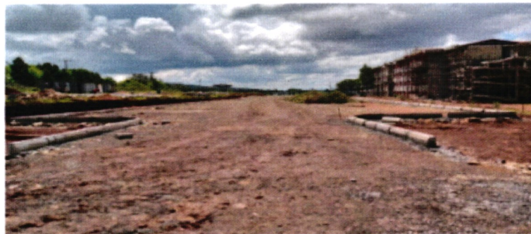
CIVIL WORKS DRIVEWAY & PARKING COMPACTED SURFACE READY TO RECEIVE CABBRO BED AND CABBRO SURFACE FINISH
