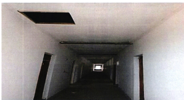
INTERIOR OF BLOCK A SCHEMING WORK
