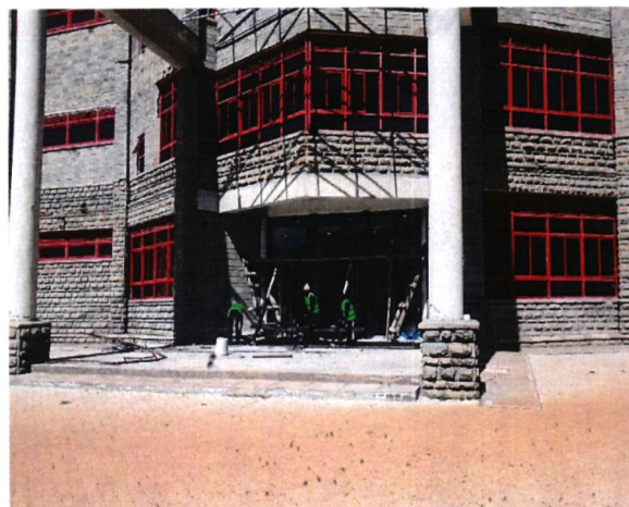
Fixing of automated basement door
