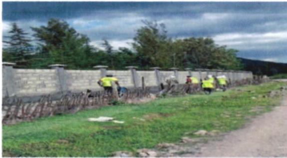
Mara primary School-Ongoing construction of a perimeter wall
