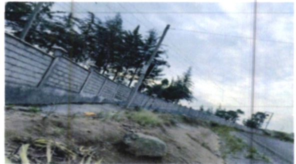
Kamahia primary School-Ongoing construction of a perimeter wall
