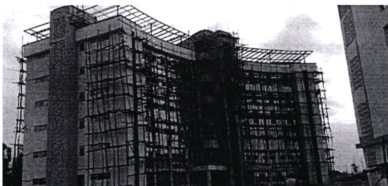
Proposed RFTITT construction on-course
