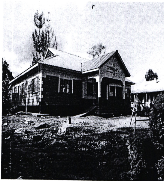
CONSTRUCTION OF AN ADMINISTRATION BLOCK AT MWANIANJAU MIXED SECONDARY SCHOOL
