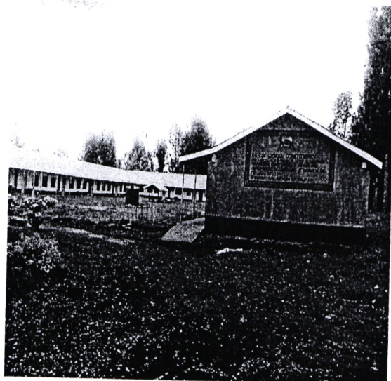
ix RENOVATION OF 16 NO CLASSROOMS AT KIAMIWATHI PRIMARY SCHOOL
