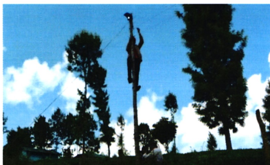
Setting up the Power Grid at Magiro Hydro
