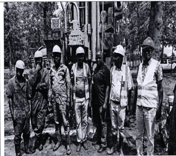
KPC Team after completing drilling of borehole at Set Kobor Primary School
