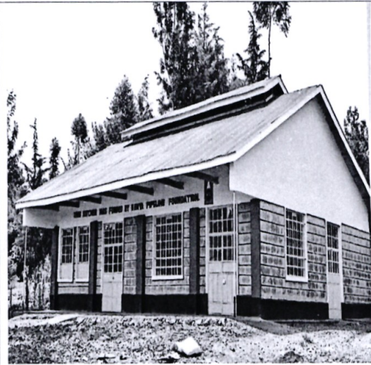
Completion Modern Kitchen at Kapchebet B Primary school
