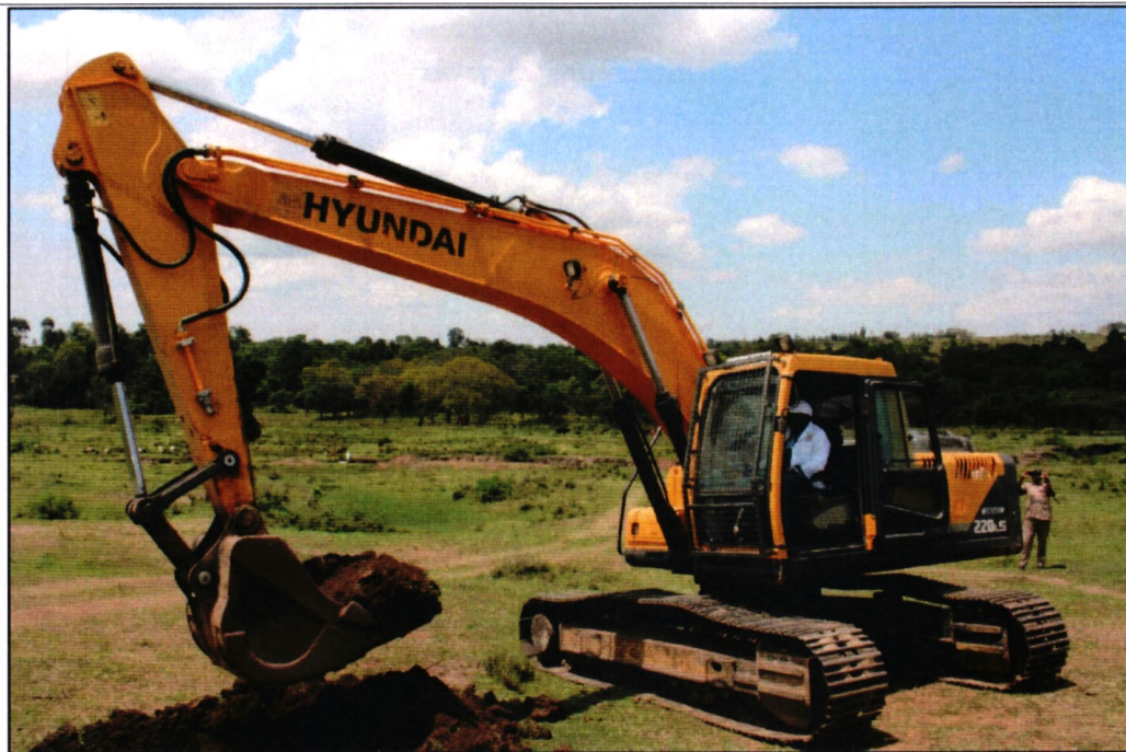
Ground breaking of the Kimintet Peace dam
