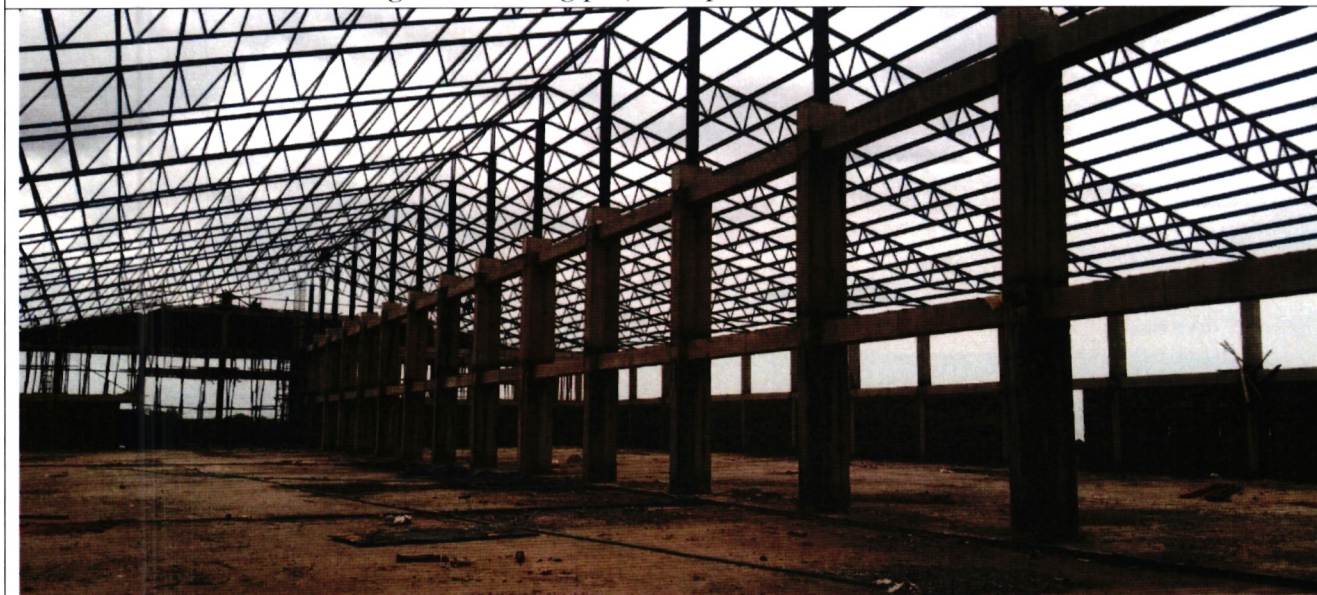
Steel structure erection in preparation for roofing.
