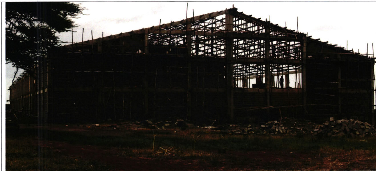
Oloitokitok Agro-Processing project super structure under construction
