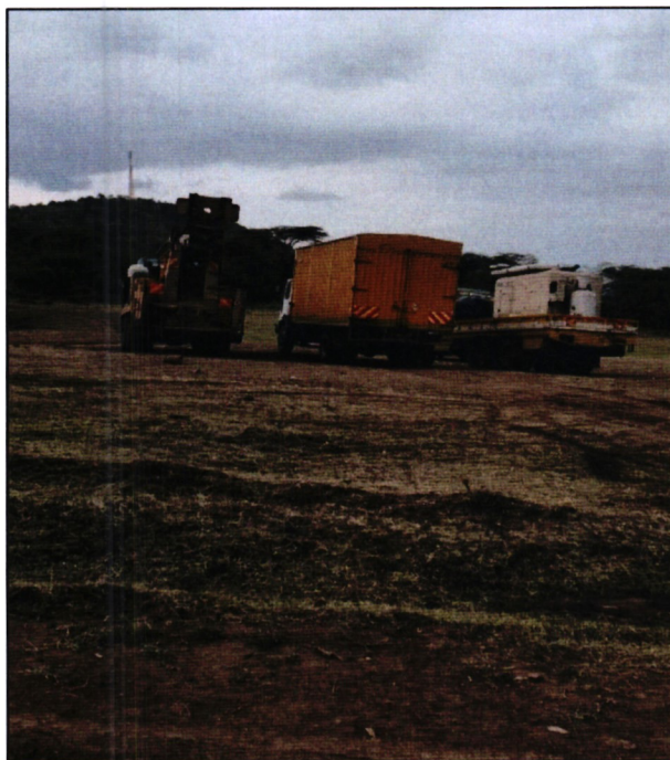
Equipment mobilization to Lemek bore hole
