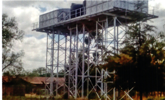
Water reticulation at Lanet in Nakuru
