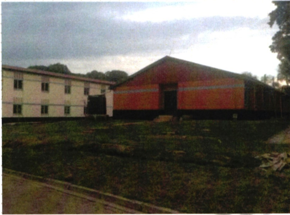
Ongoing renovation of hostels
