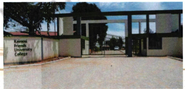
Gate, Road works and Associated Works
