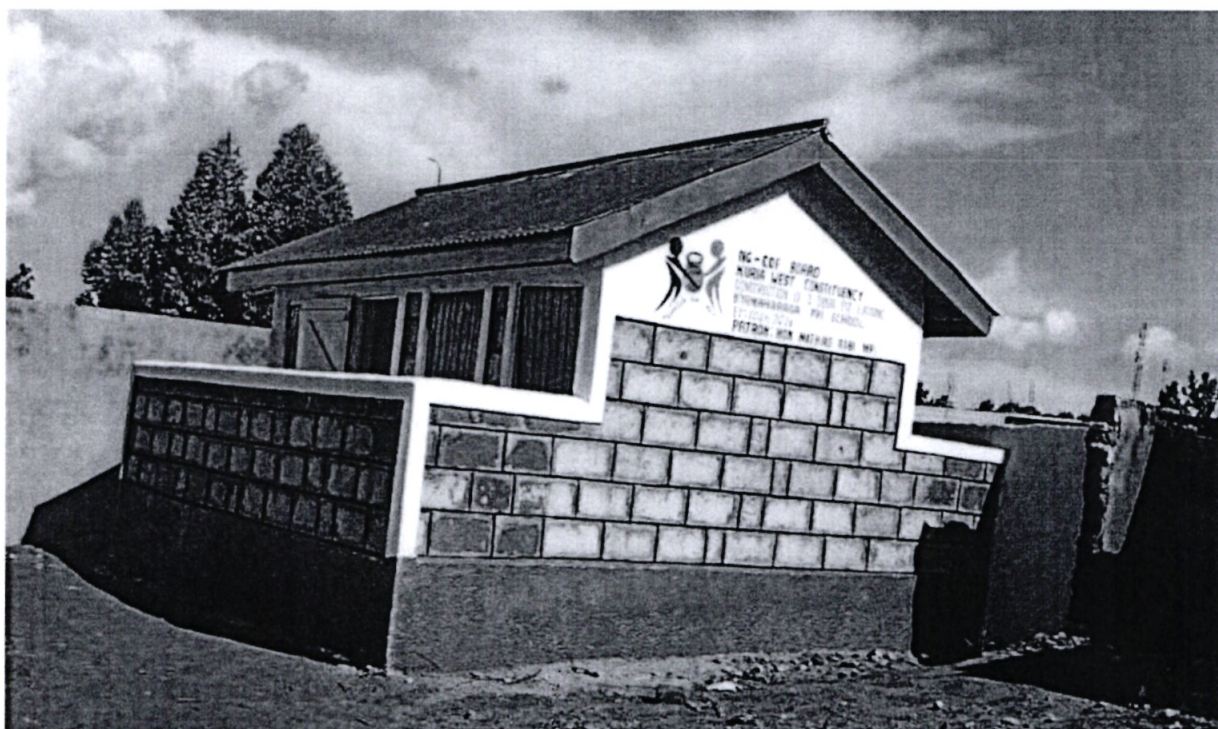
NYAMAHARAGA PRIMARY SCHOOL –Construction of 8 door Pit Latrine at Kshs 800,000
