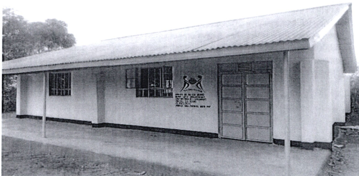
BIAMITI PRIMARY SCHOOL- Construction of 1 no. classroom at Ksh 952,734
