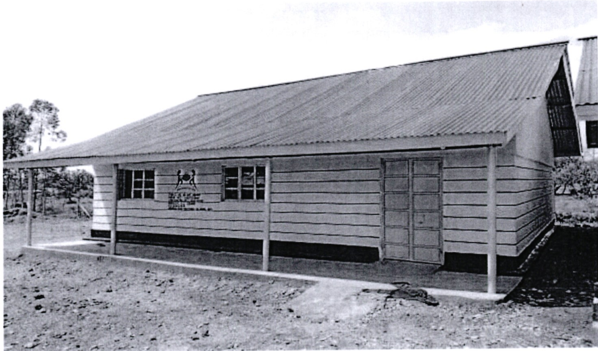
Nyaiqutu Primary school; Construction of 1 no. classroom
