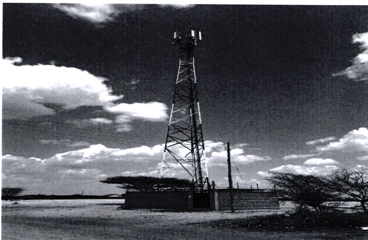
Bisan Biliqu sub-location in Isiolo North, strengthening Kenya's broadcasting and telecommunications sector.
