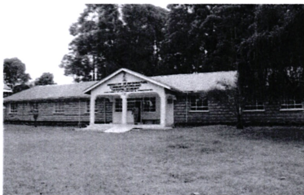
Information office KNA modernization Eldoret Uasin Gishu County.
