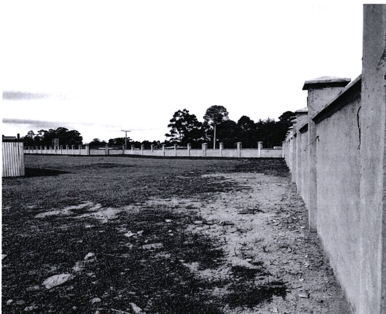
Perimeter wall for KIMC Eldoret campus at Kiamba.
