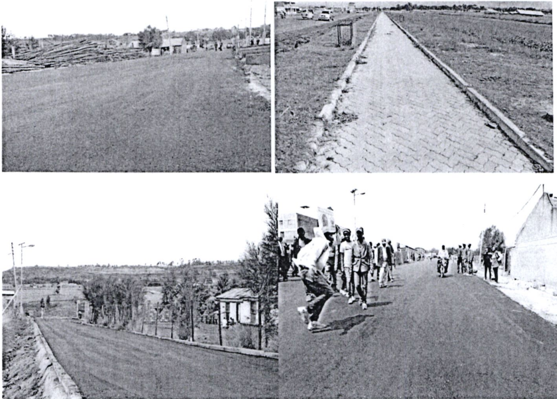
Bitumen Works, Paved Pedestrian Parhways
