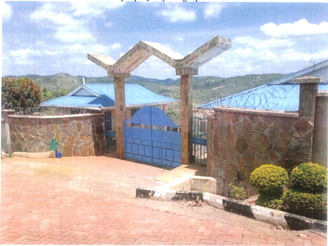
Photo 1. A section of Murang'a project- Main entry
