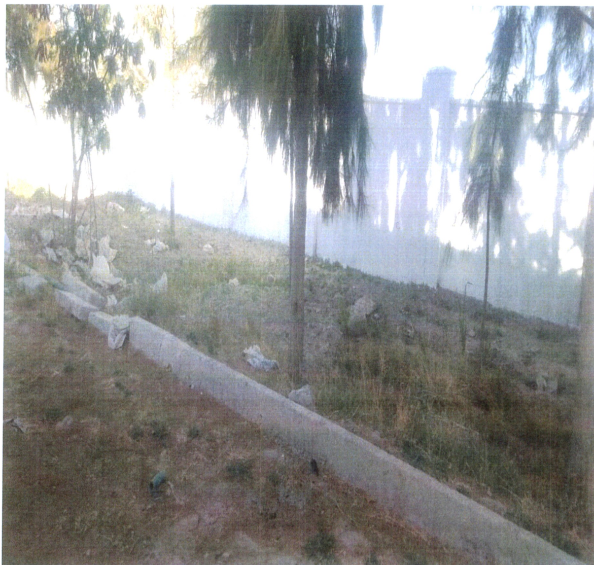
Photo 6: CWSK Integrated child and family centre - Joska – A section of perimeter wall - complete
