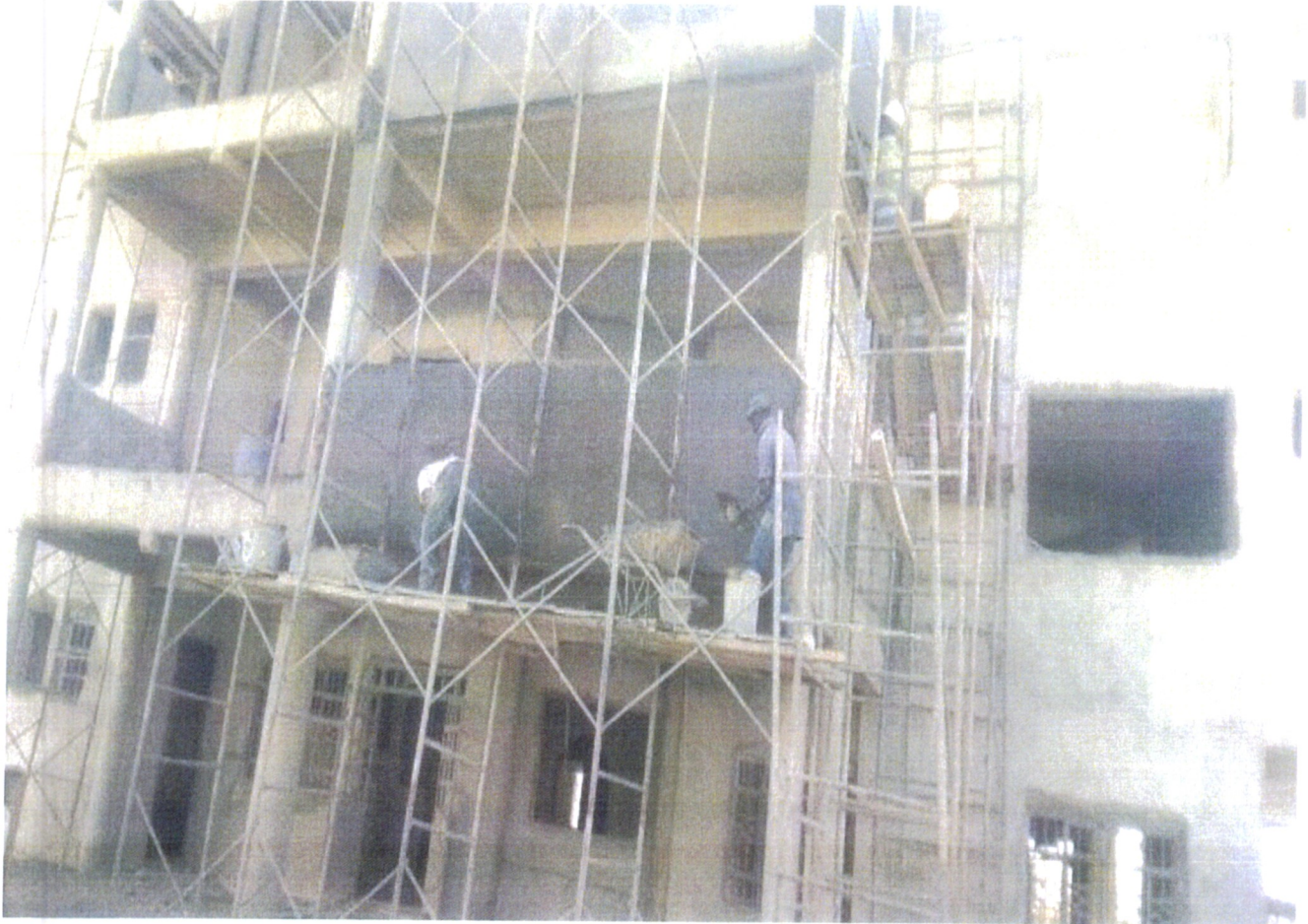
Photo7: CWSK Integrated child and family centre - Joska – A section of Maisonette 3 work in progress
