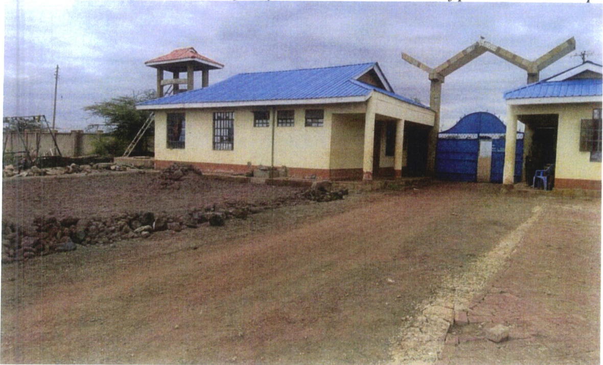
Photo 7: CWSK Integrated child and family centre - Isiolo – Health centre and guard house units complete
