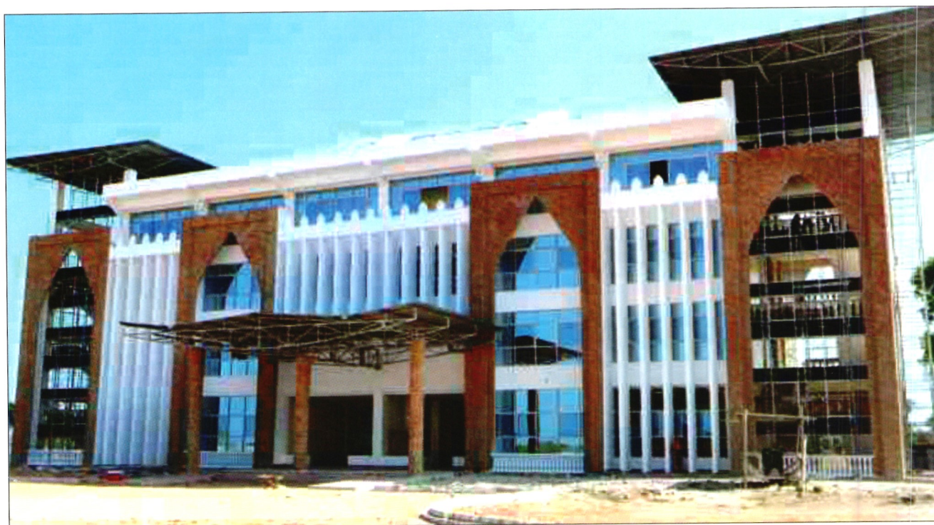
Lamu port office block nearing completion
