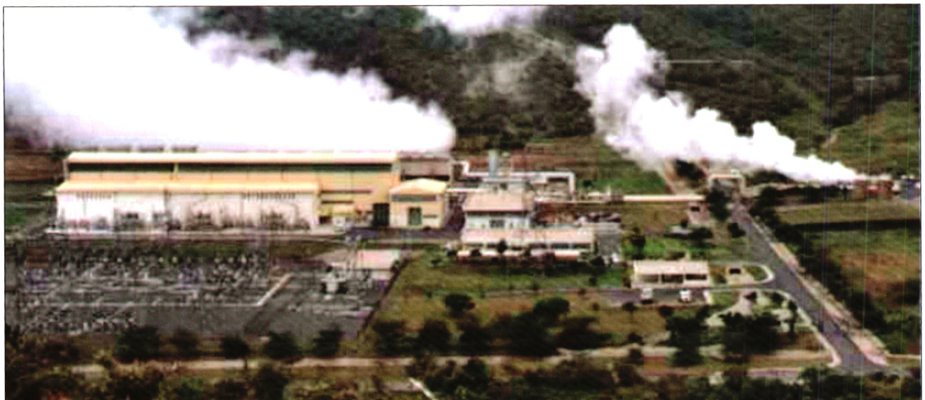
Olkaria geothermal power plant
