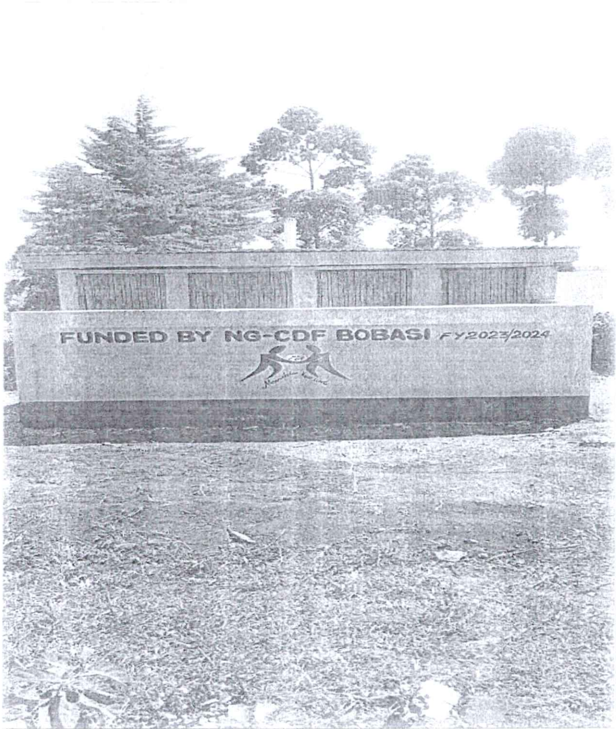
Fig. 2 EBIGOGO PRIMARY SCHOOL – Construction of 4 door pit latrine
