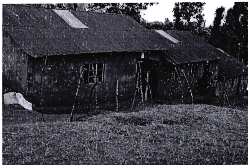
Fig. 1.0–Renovation of 6 No. classrooms at Gitwe Primary School (FY 2024-2025)
