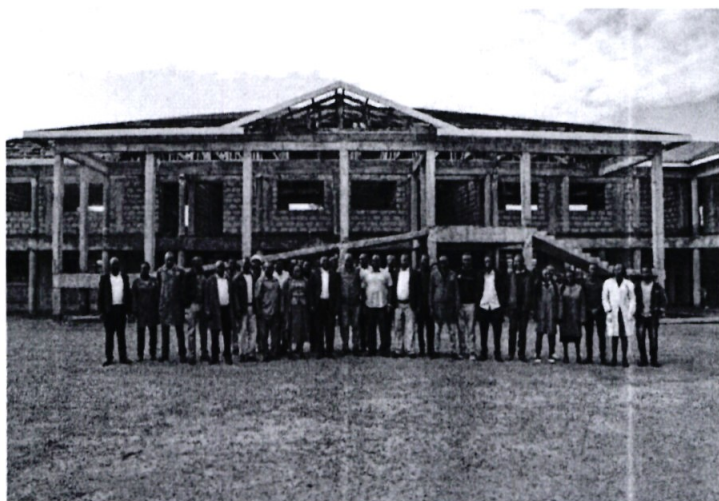
Ongoing construction of Storey tuition block at sergoit primary school
