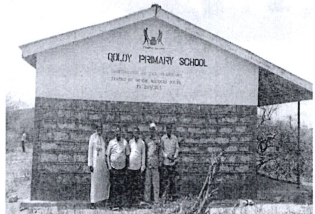
QOLOY PRIMARY SCHOOL CONSTRUCTION OF 2NO. CLASSROOMS FY 2024/2025
