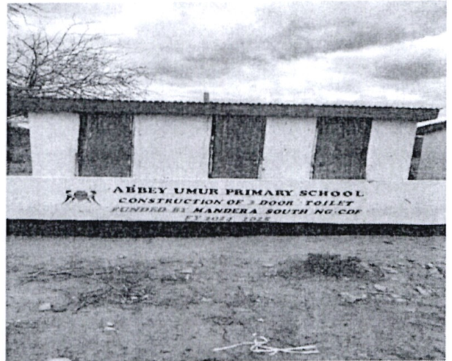
ABBAY UMUR PRIMARY SCHOOL CONSTRUCTION OF 2NO. DOOR TOILETS FY 2024/2025
