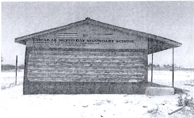
TAWAKAL MIXED DAY SECONDARY SCHOOL RENOVATION OF CLASSROOMS FY 2024/2025
