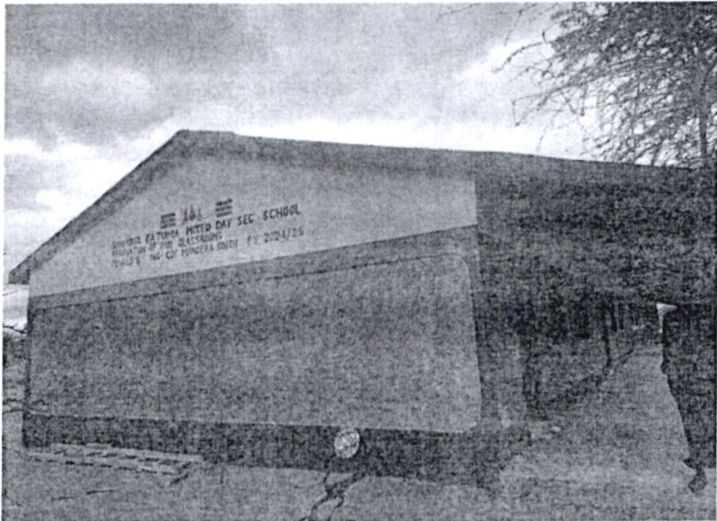
SHIMBIR FATUMA MIXED DAY SEC SCHOOL RENOVATION OF 2NO. CLASSROOMS FY 2024/2025
