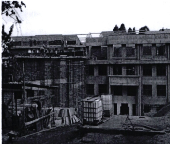
Figure 11(a): Front view of Tuition Block Phase II
