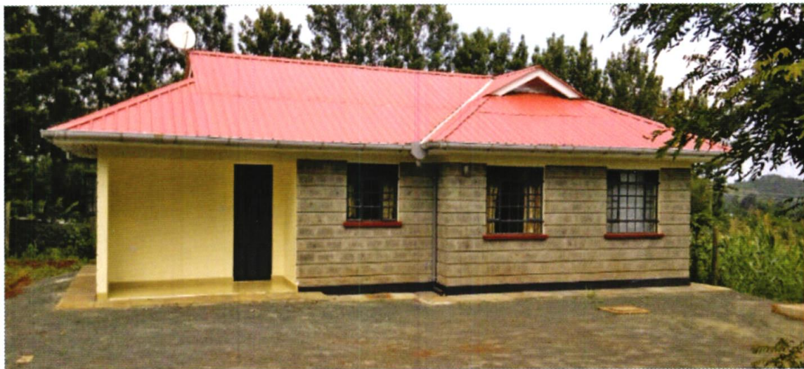
IPOA Photo 8: A Pilot Modern house for senior police officers at Sagana Police Station which was launched by the PS Interior & Coordination of National Government.
