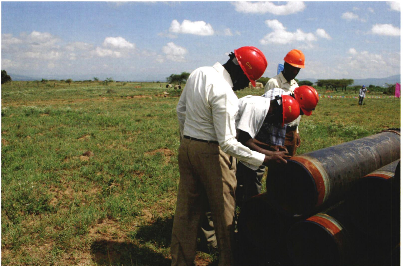
KPC engineer checking on integrity of pipeline
