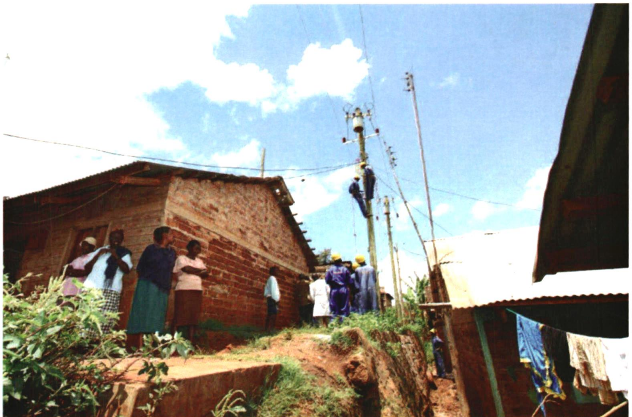
Kenya Power technicians prepare to install electricity to a house in Majimbo, an informal settlement in Embu County in April 2013.
