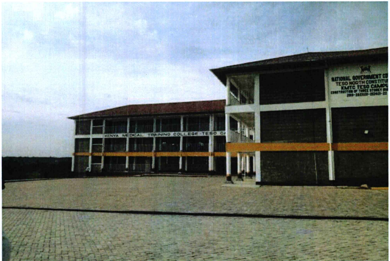
Construction of a 2-storey building to completion Kmtc Teso campus
