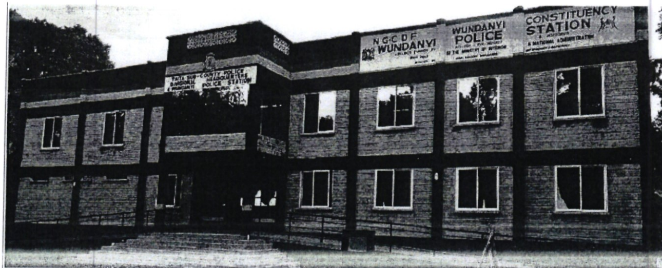
CONSTRUCTION OF MODERN TAITA SUB-COUNTY HEADQUARTERS & WUNDANYI POLICE STATION
