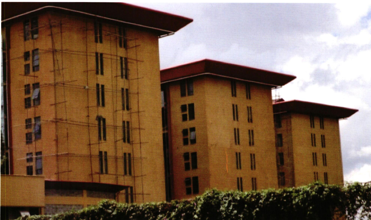
The New Mitihani House (Ongoing Project)
