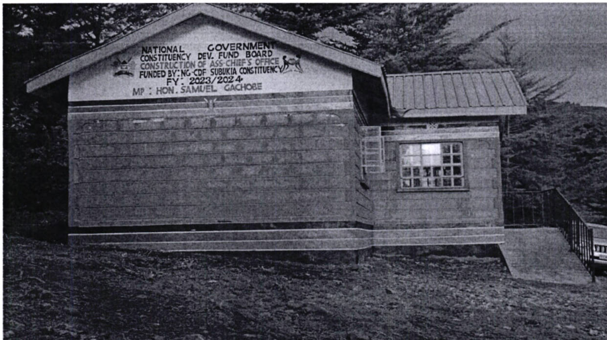
Kianoe Chiefs Office – Construction of Asst. Chiefs Office
