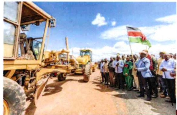
Launching of the construction of the Ngoswani-Morijo Road in Narok County
