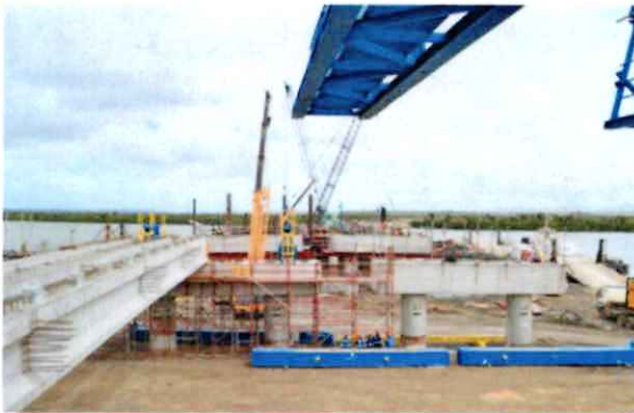
Mwache junction-Tsunza-Mteza road under construction
