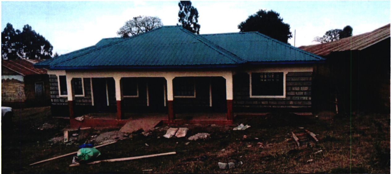
Murangine Primary School Construction of Administration Block done in FY 2019/2020
